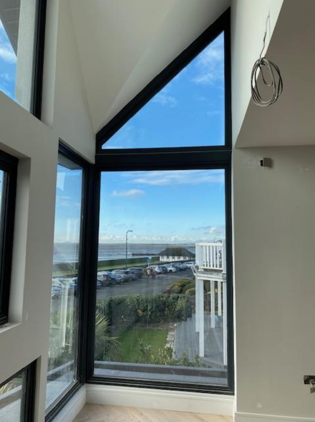
View from ff flank window west toward No.73
